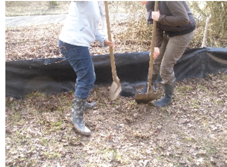
Illustration 5: Installation du barrage
